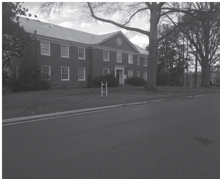
Eggleston Hall will soon be brought down. Photo Credit: Jonathan Walkey
